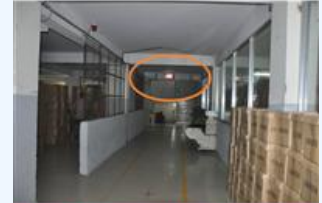
No backed up power emergency light has installed to illuminate the egress corridor during emergency
