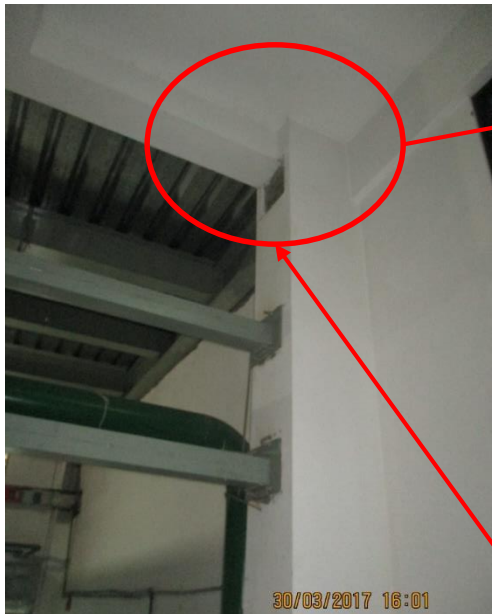
RC beam column system of South side Stair
