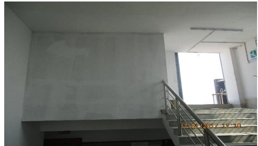
Bottom slab of OHWT
