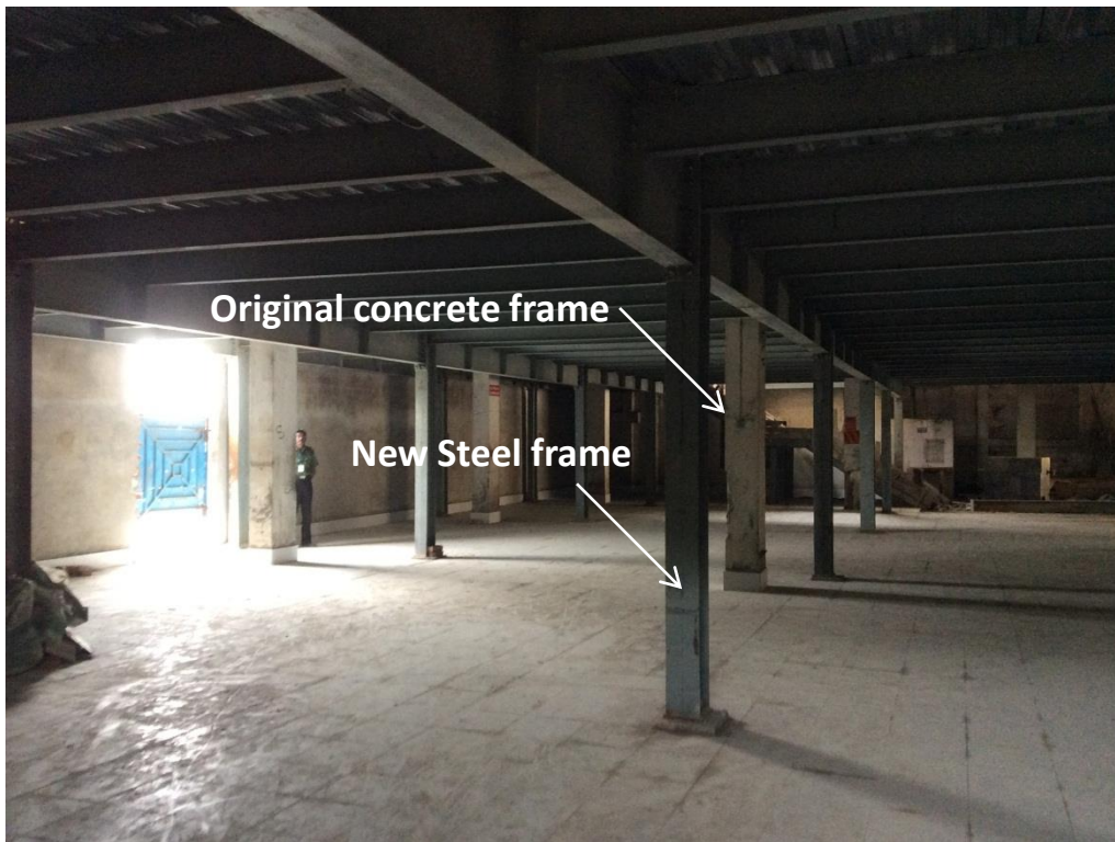
Original Shed with new steel mezzanine infill.
