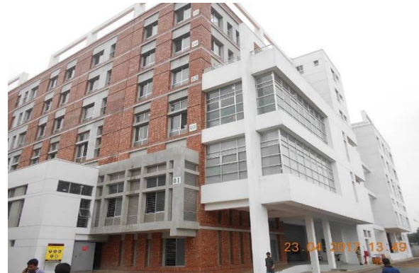
East Side of The Factory Building
