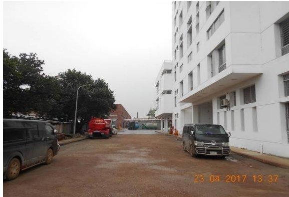
South Side of The Factory Building
