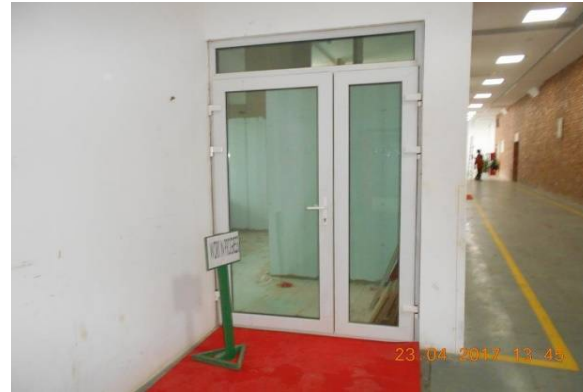
Child-care Room (Under Construction)
