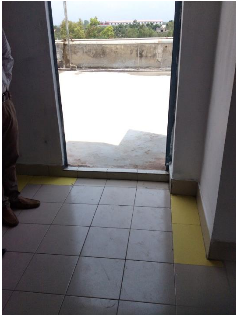
65mm Build Up at roof Level
