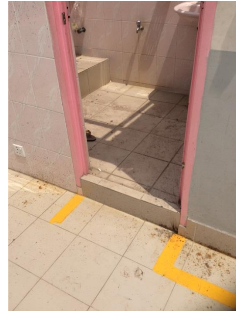
Additional 90mm Build Up In toilet area at roof level.
