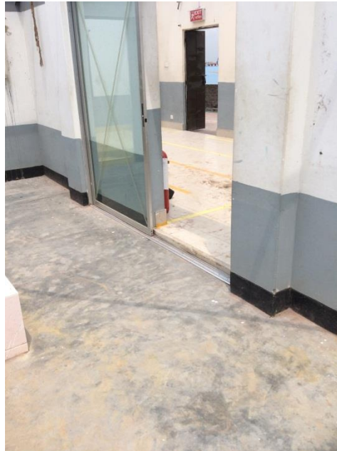
Additional 60mm Build Up at roof Level
