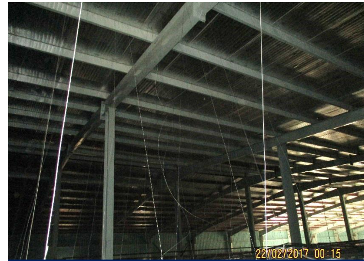
Missing bracing
