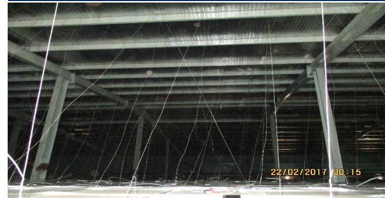
Missing bracing
