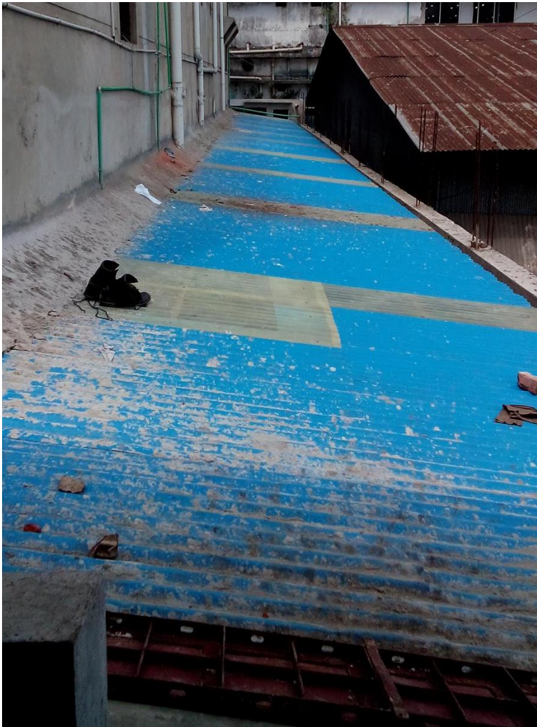
Mono-pitched roof lean to the production building
