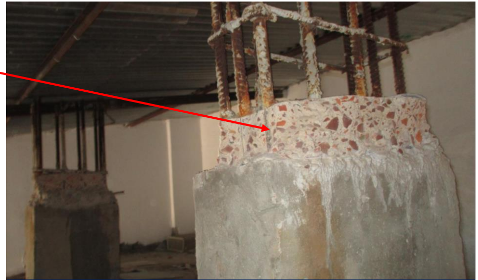
10 numbers of rebar found on column C5
