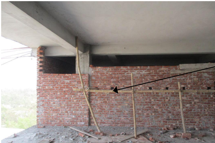
Internal 5" brick walls not shown in as-built drawings
