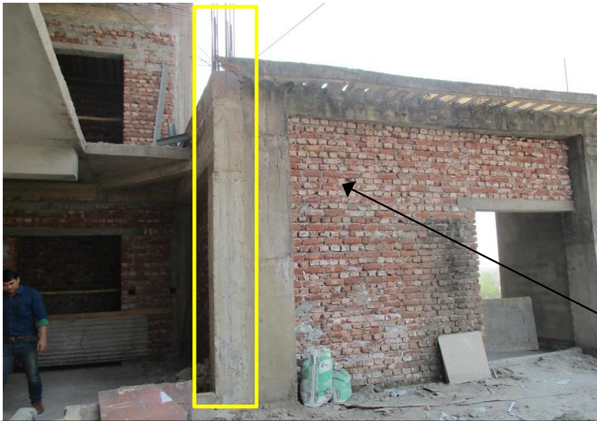
Additional RC column with 12 number of rebar
