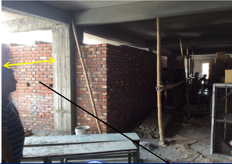
Toilet Build-up and Brick Partitions on Cantilever
