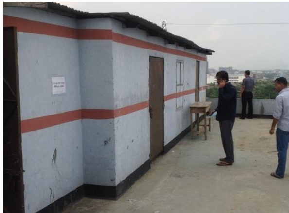
Maintenance Room to East of Building 1 at Roof level
