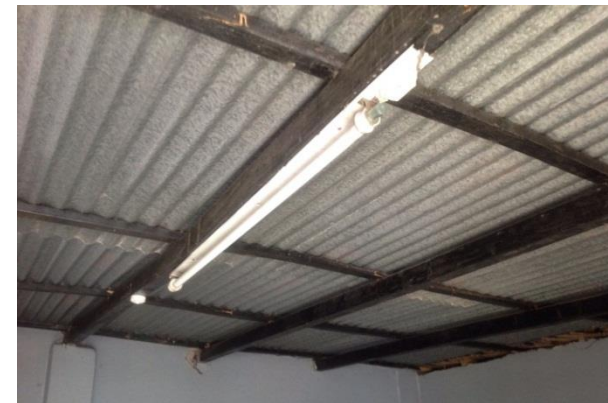
Roof to Maintenance Room
