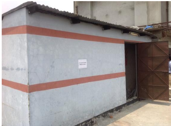
Maintenance Room to West of Building 1 at Roof level
