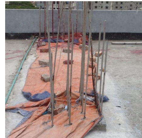
HY rebar at Roof level
