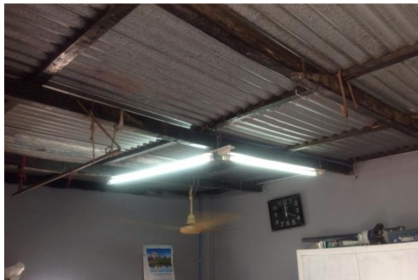
Roof to Maintenance Room
