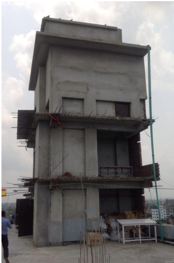
Water tank above stair core of Building 1
