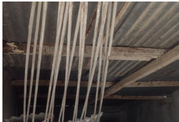
Lightweight roof to stair core
