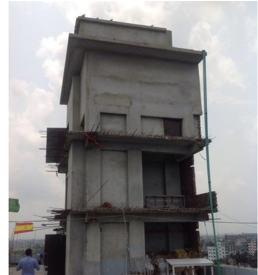
Two additional floors to stair core to West of Building 1
