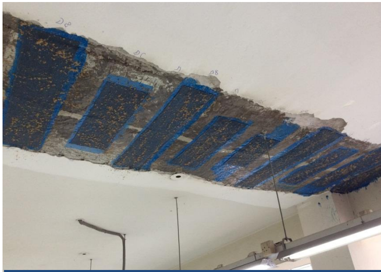
Repairs to cracking on soffit of 5 th floor
