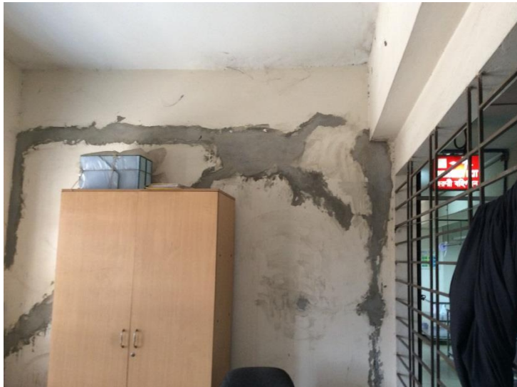
Cracking in internal brickwork wall
