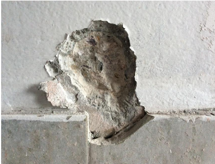
Stone aggregate visible in column at G Floor
