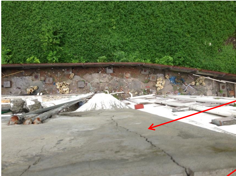
Uncontrolled cracking MJ in façade
