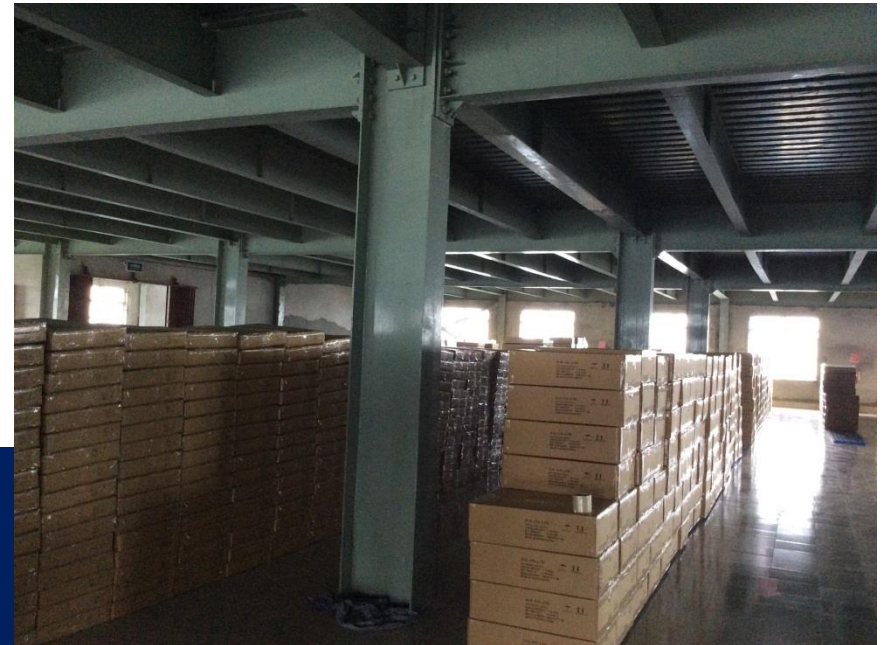
Warehouse loading on GL, L2, and L3
