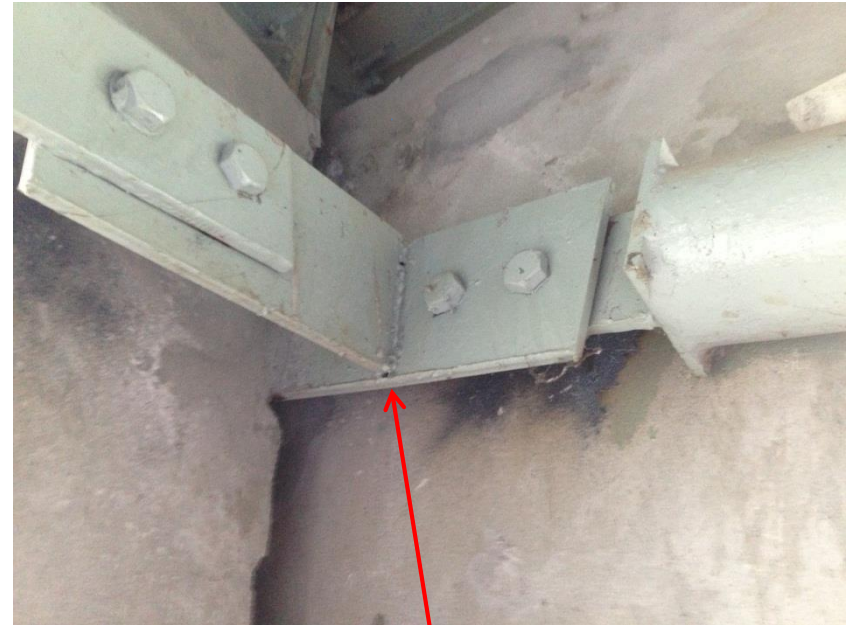
Bracing welded onto gusset plate of bracing in orthogonal direction
