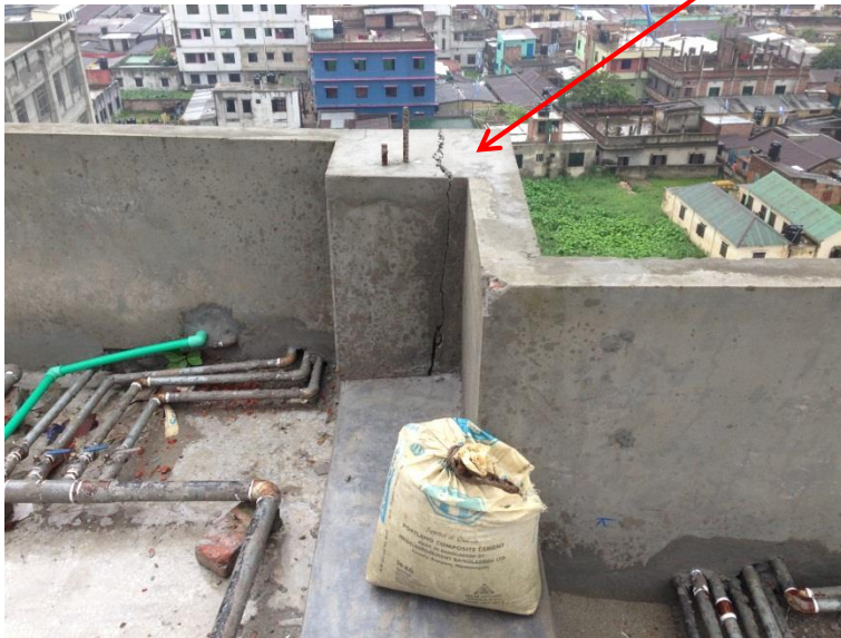
Uncontrolled cracking MJ in façade
