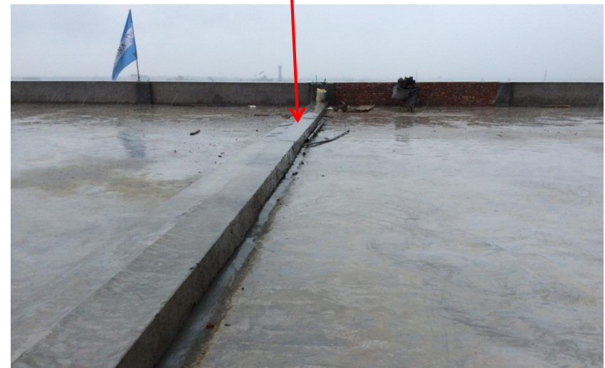
Highlighted area indicates movement joint
