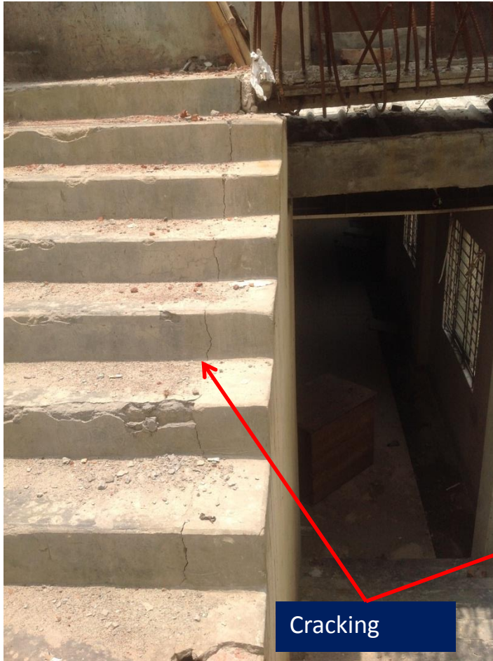
Cracking of stairs
