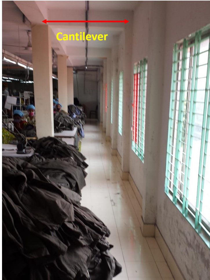
Cantilever on South elevation (internal view)
