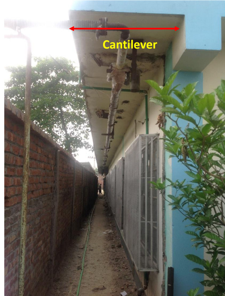
Cantilever on South elevation (external view)
