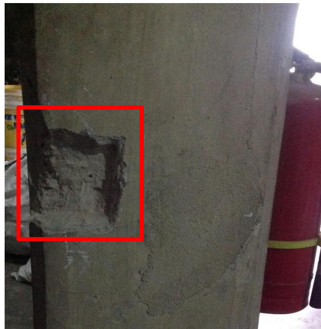
Tested Ground Floor Column – Brick Chips
