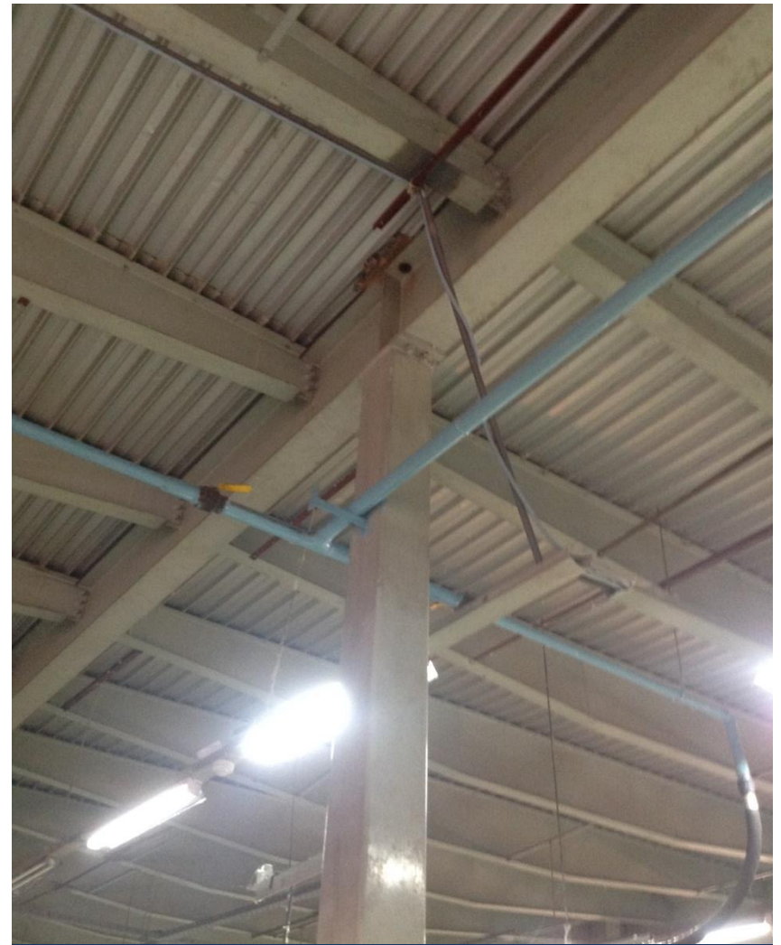
Soffit of metal deck floor (Knitting house)
