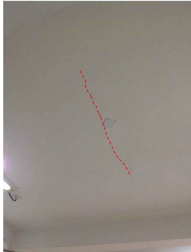
Soffit of roof slab
