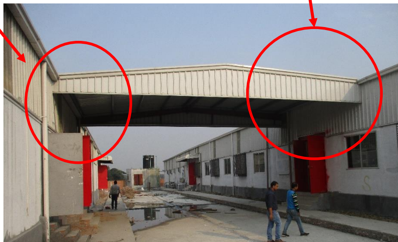
Canopy between Tin Shed-3 and Tin Shed-4
