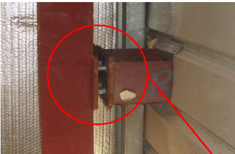
Canopy connects with Tin Shed-4
