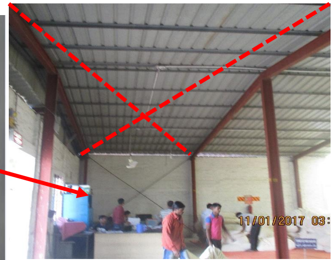
Vertical bracing of 20 mm diameter rebar
