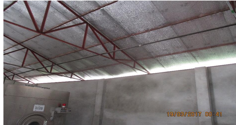
Inadequate connection between truss and brick walls (Shed#2)
