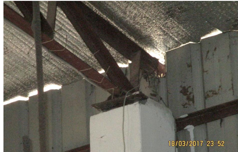
Poor Connection between RCC column support and truss connections(Shed#1)
