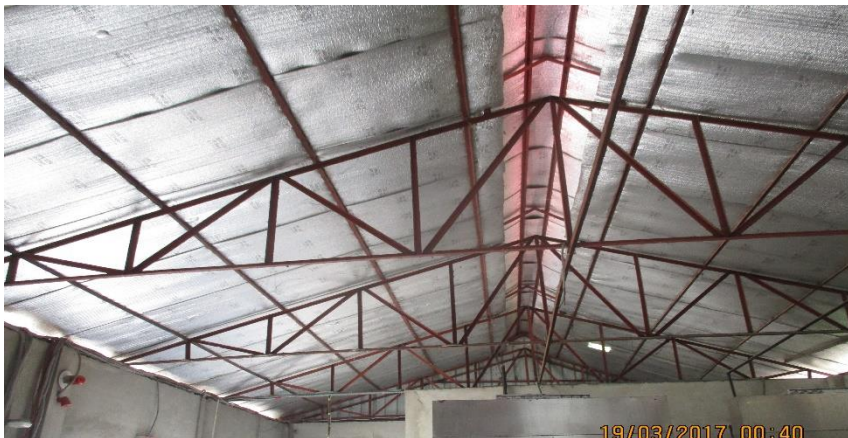
No lateral system were observed to resist lateral loading (Shed#2)
