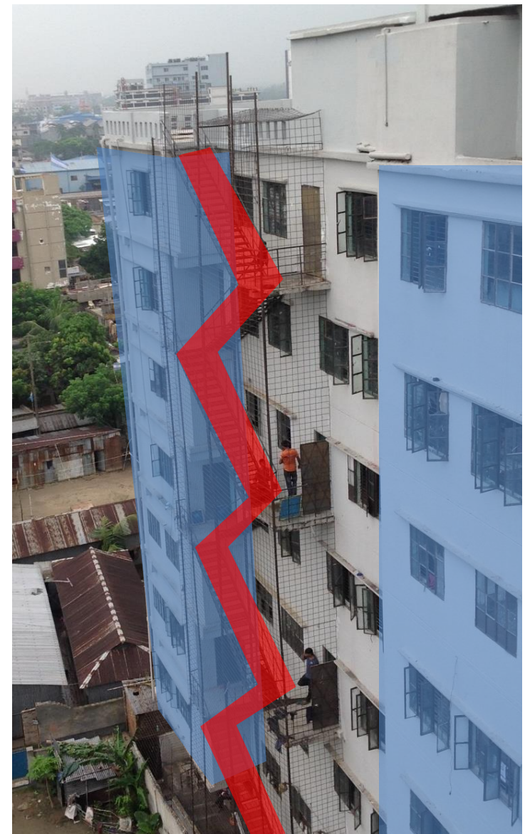
Steel escape stairs and cantilever structure to the south of E-W Building
