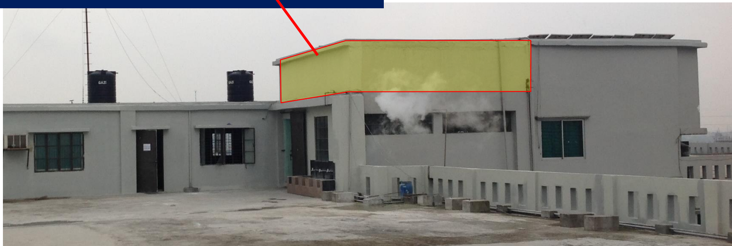
Concrete water tank
