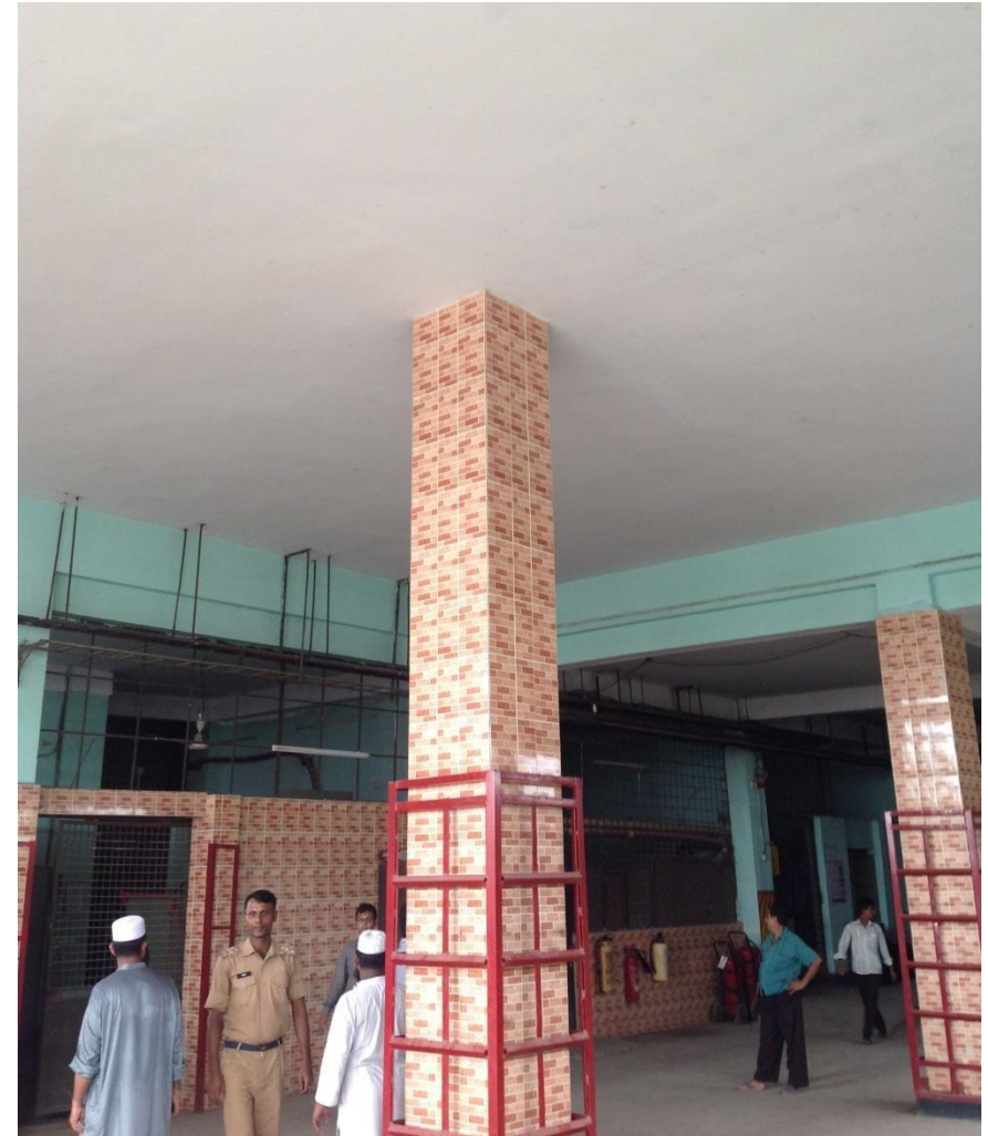
Angle steel frames at columns
