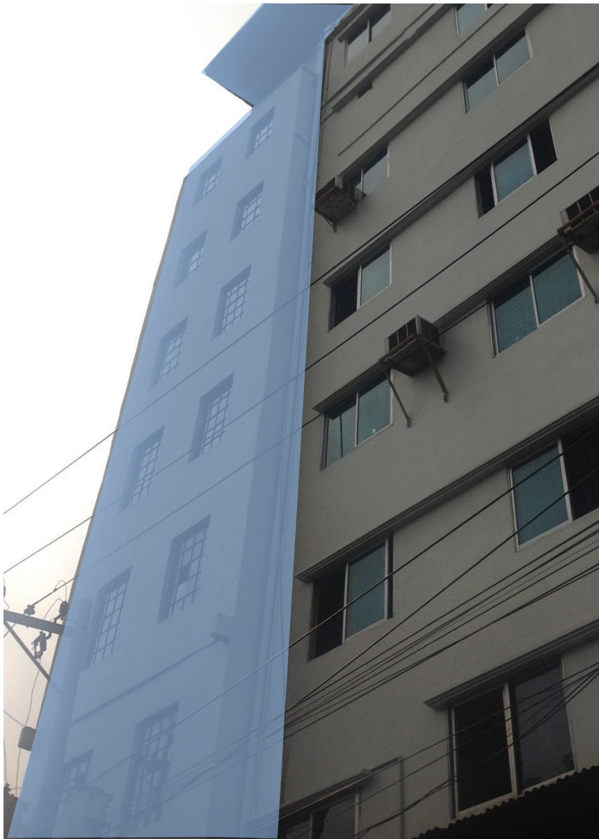
Cantilever structure to North of N-S Building
