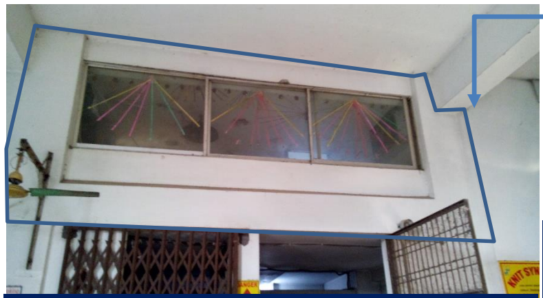
Mezzanine floor at ground level
