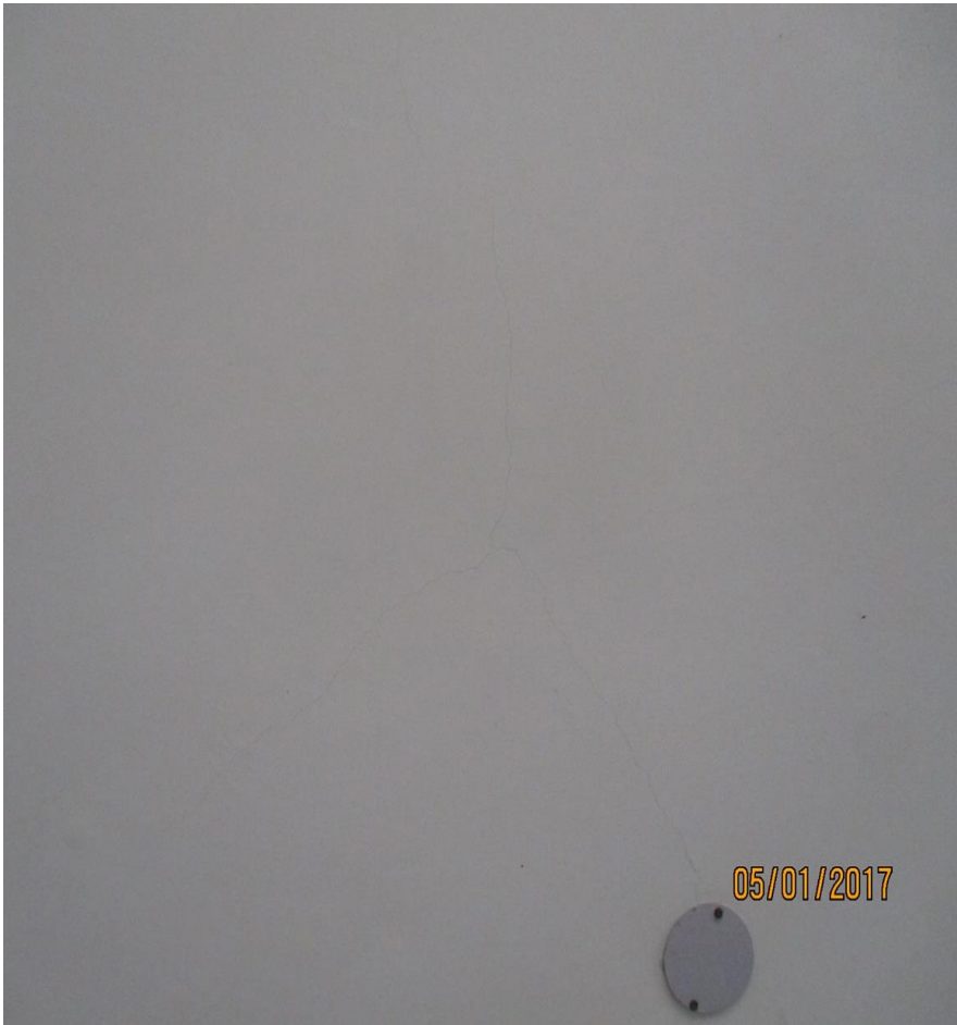
Hairline cracking observed on beam and slab at 5 th floor level
