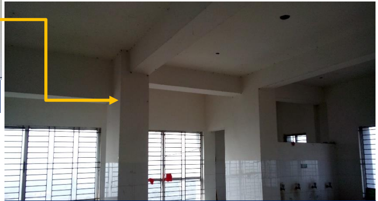
Beam with different size at west side of building
