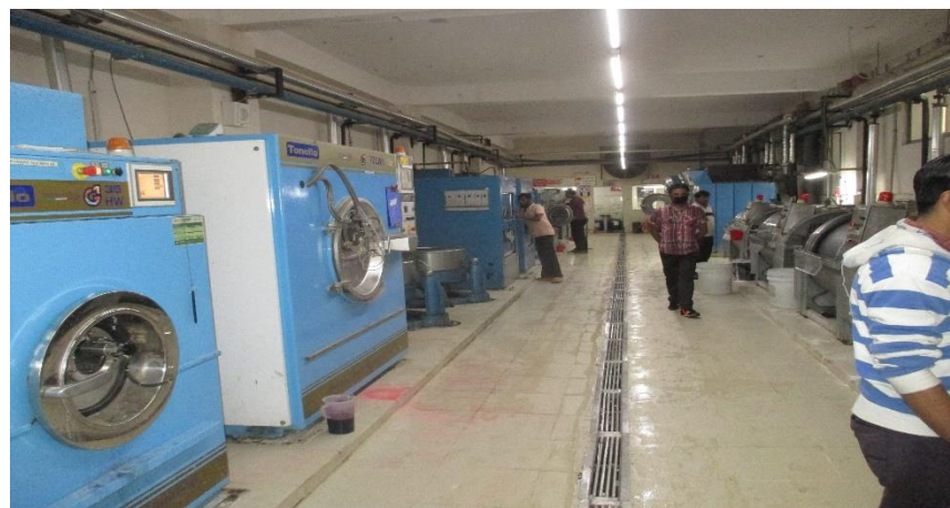
Washing area of Ground floor
