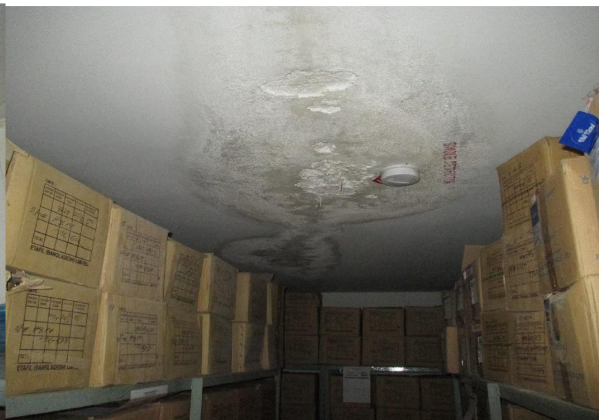
Water ingress at basement through Ground Floor slab
