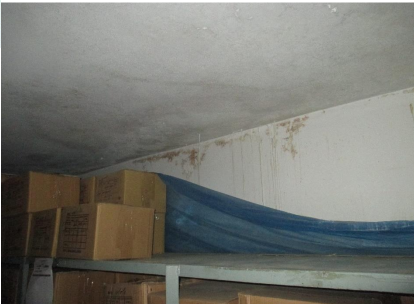
Water ingress at basement through Ground Floor slab
