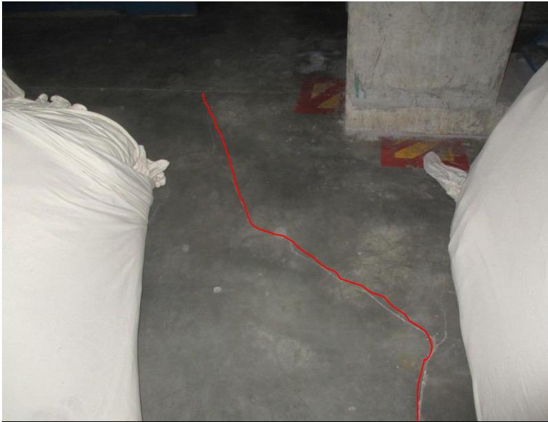
Hairline crack on slab
