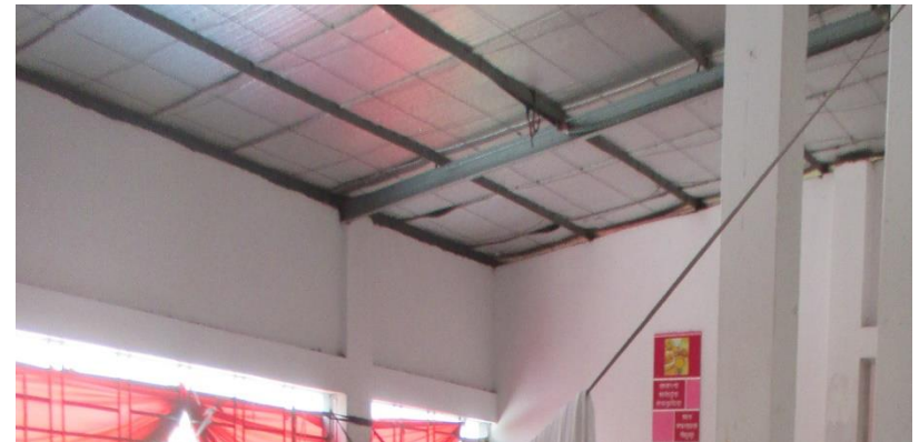
Non engineered roof (Extended portion)
