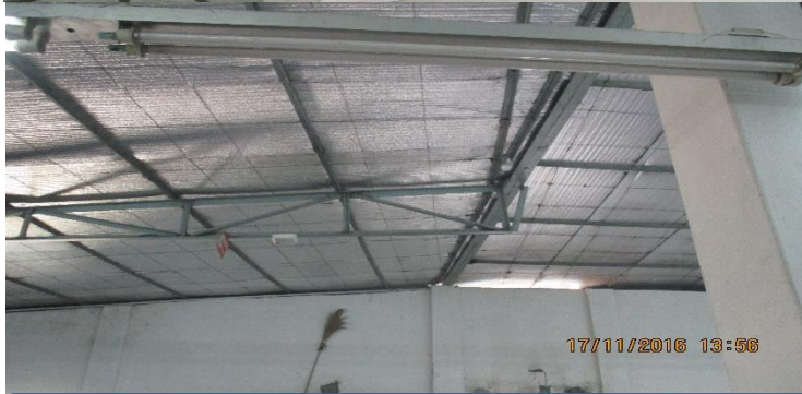
Non engineered connection (Finishing and Cutting Section, Production Shed)
