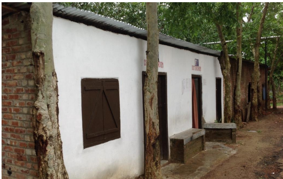
Welfare Shed – Corrugated roof on timber purlins
