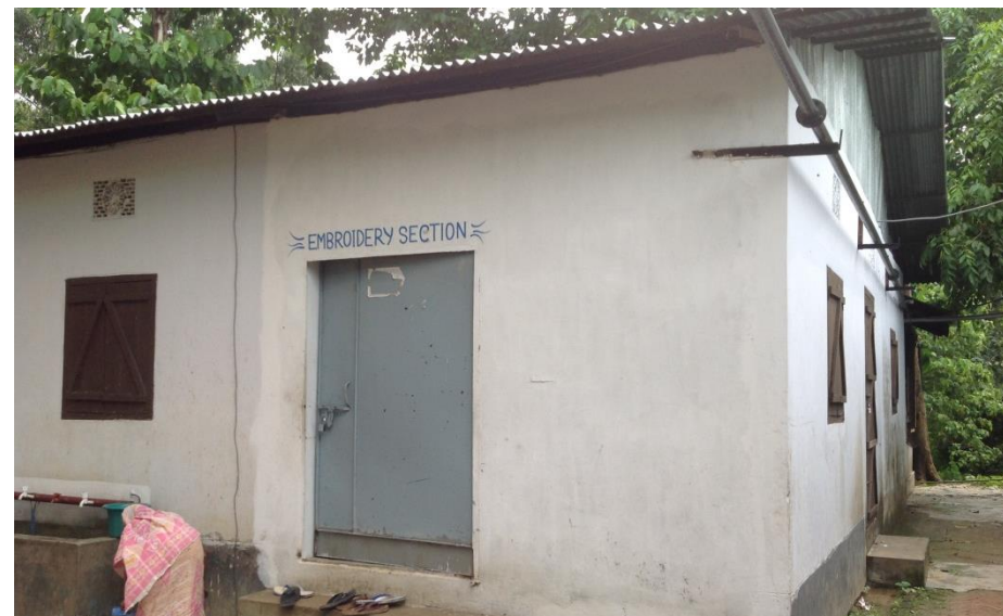
Embroidery building – corrugated roof on timber purlins
