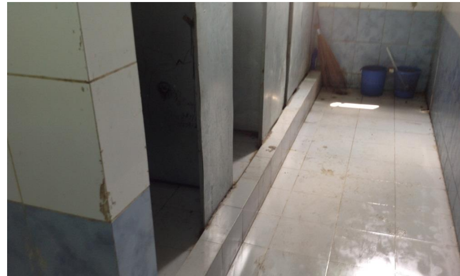
Toilet build-up at all floor levels
