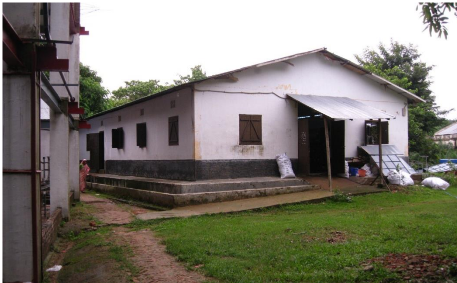
Winding building - corrugated roof on timber purlins
