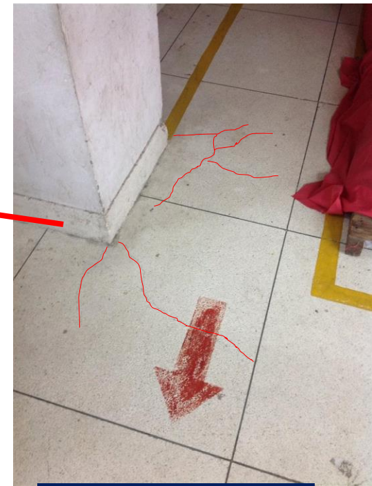
Ground Floor Slab
