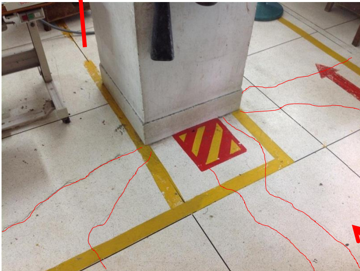
2nd Floor Slab
