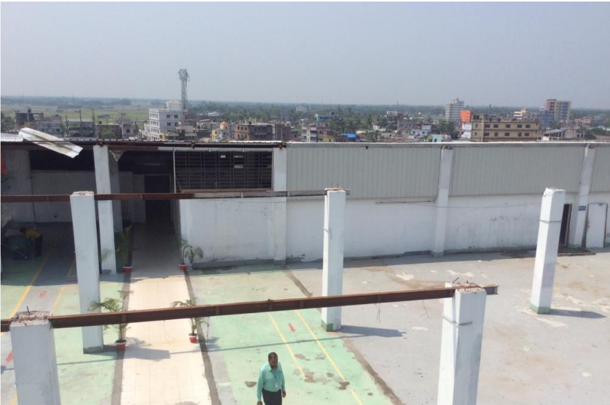
Main Building Roof
