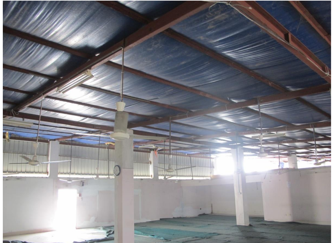
Steel work over Prayer room: Roof of Main Building
