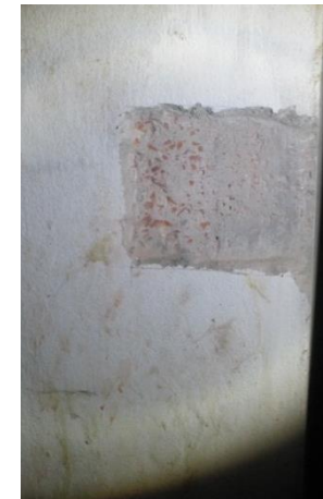
Tested Ground Floor Columns – Brick Aggregate
