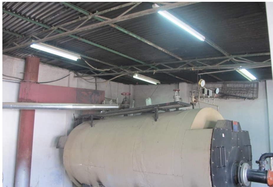
Steel work over Boiler room: Shed 3
