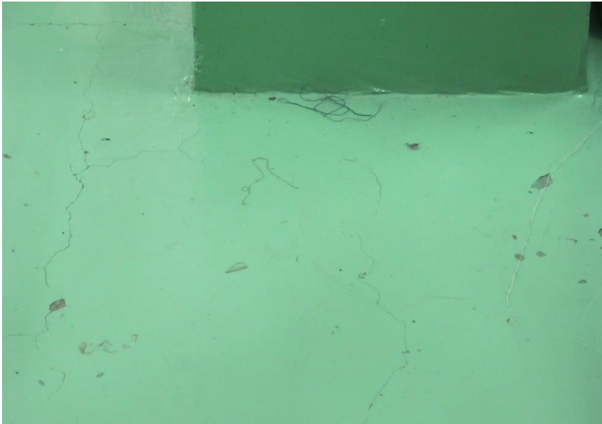
Slab Cracking Around Column Perimeter
