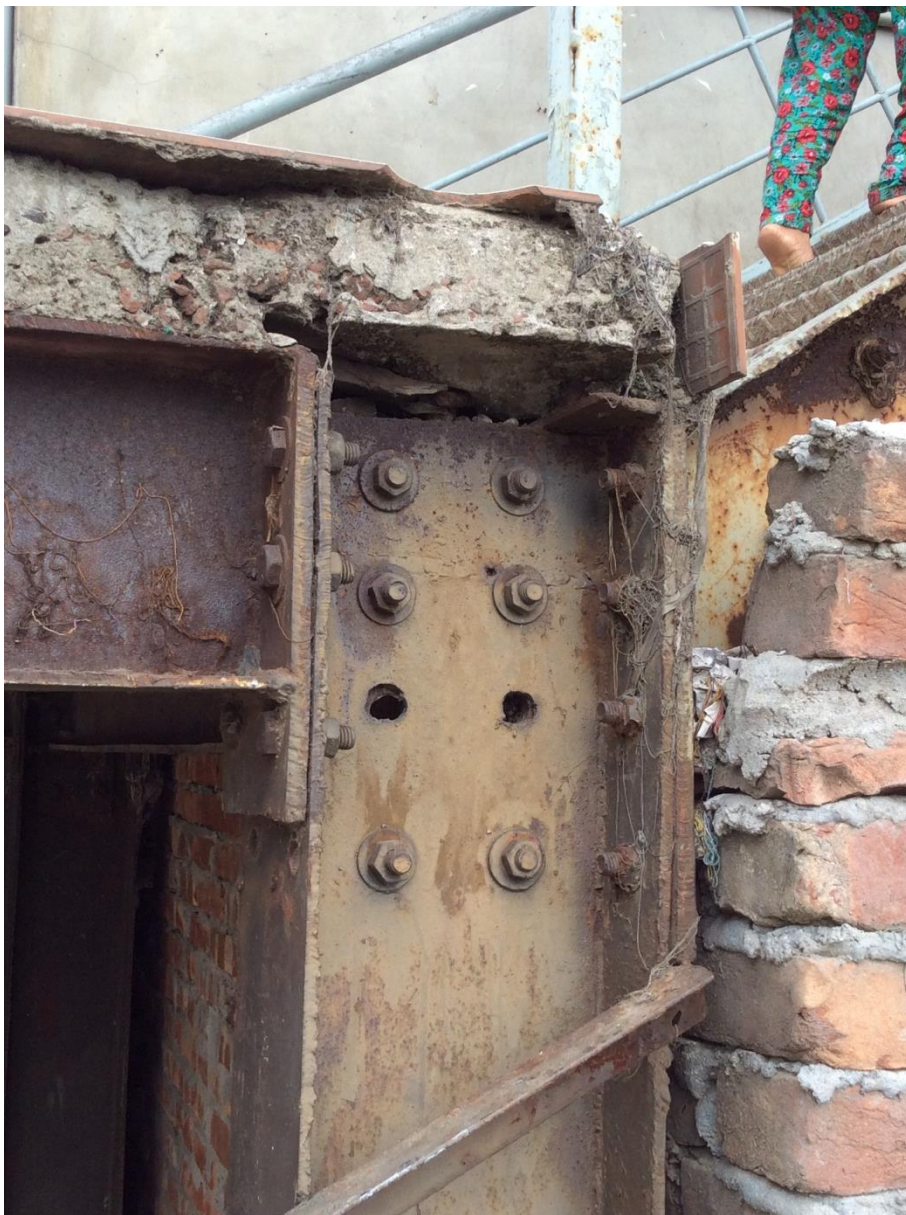
Poor connections
