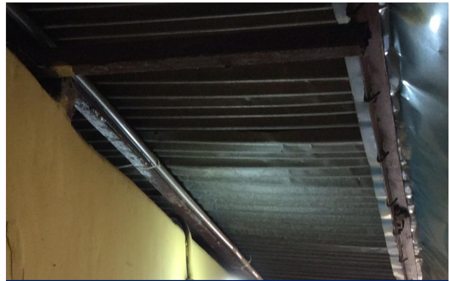
Washrooms - Corrugated roof on steel angles
