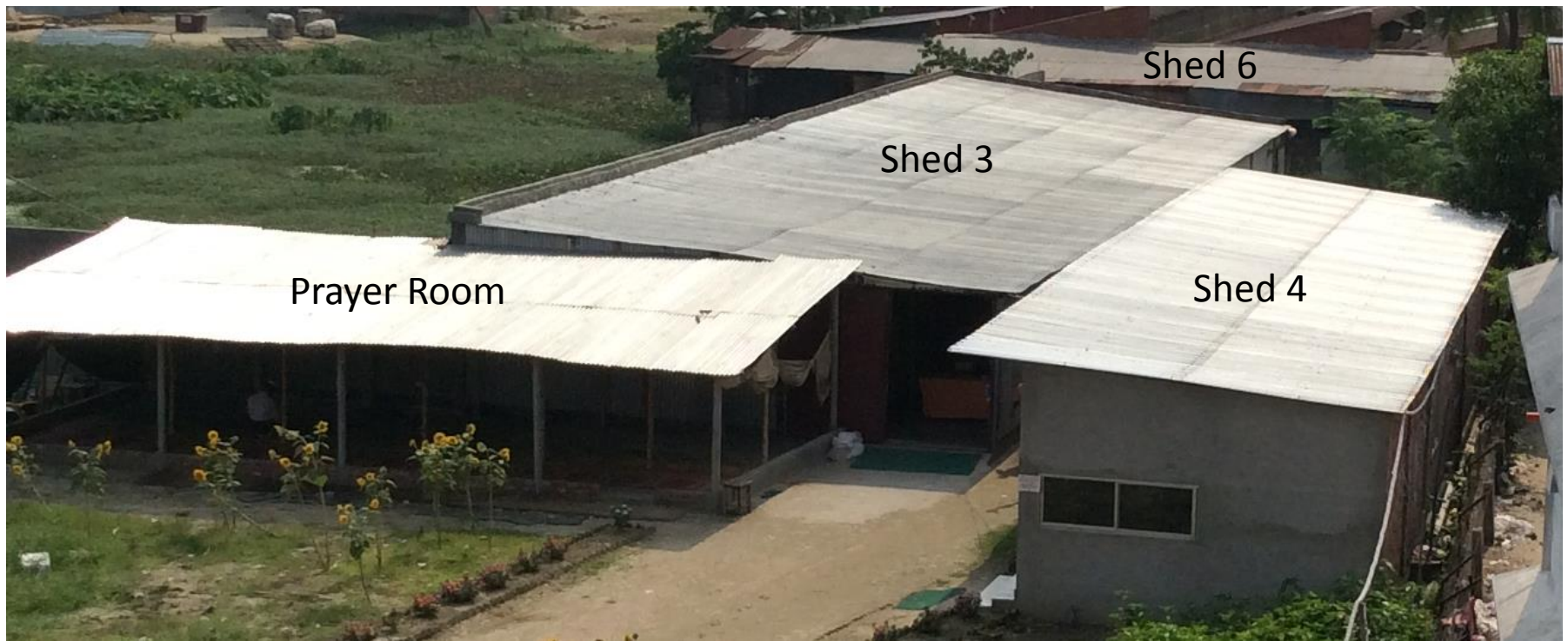
Prayer room, Shed 3 (Main Storage Shed), Shed 4 (Welfare Building), and Shed 6 (Leftover Fabric Storage Shed)
