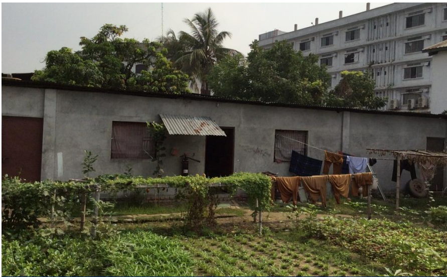
Shed 5 – Corrugated roof on steel angles on masonry walls
