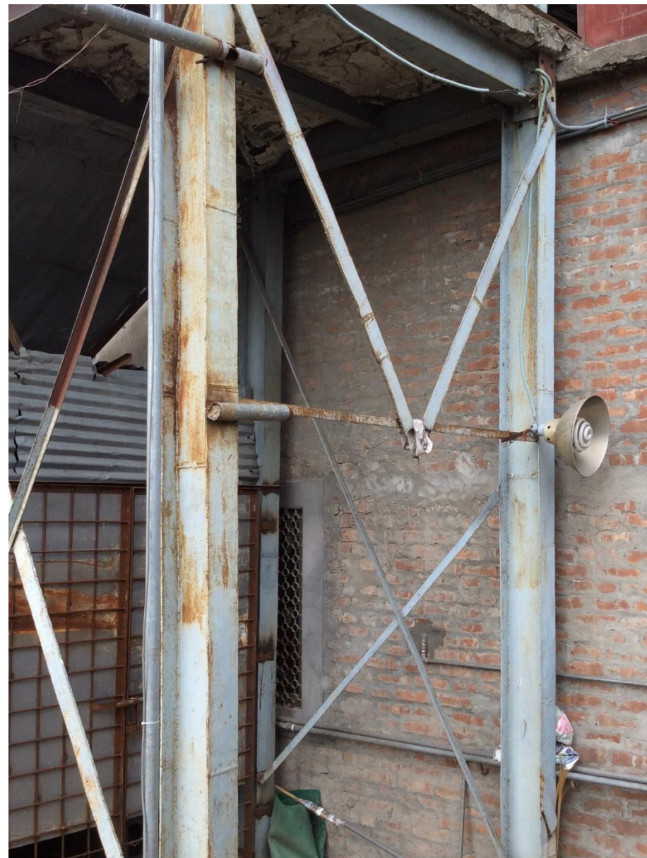
Inadequate bracing
