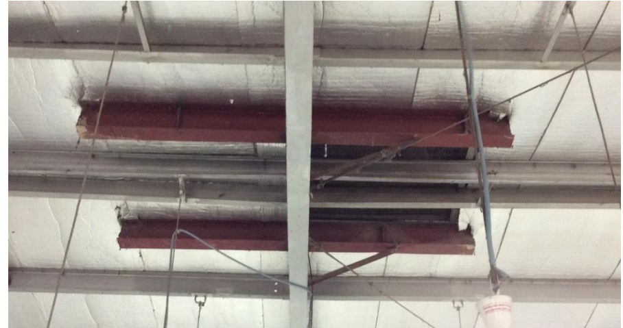
Connection detail unclear – single bracing member only
