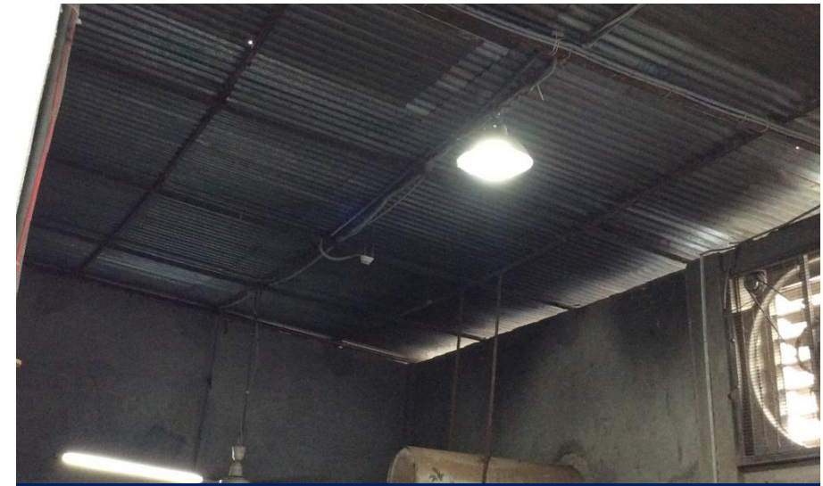
Generator Room – Corrugated roof on steel angles
