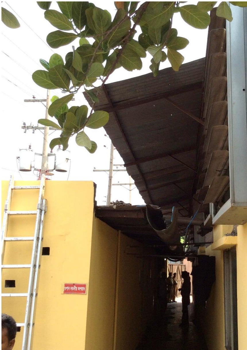
Washrooms and canopy to Shed 2
