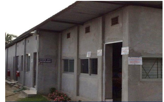
Shed 4 – Corrugated roof on steel angles on Masonry walls
