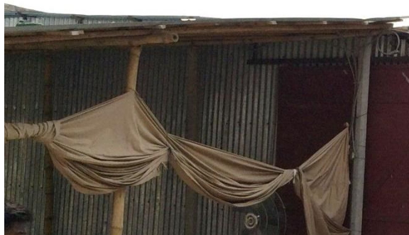
Prayer Room – Corrugated roof on bamboo purlins & posts
