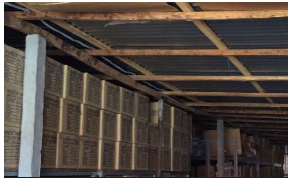
Shed 3 – Corrugated roof on timber purlins on concrete posts
