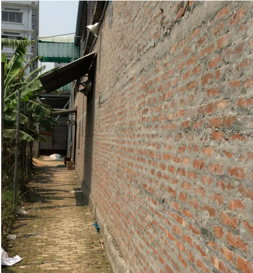
Masonry wall to Shed 2
