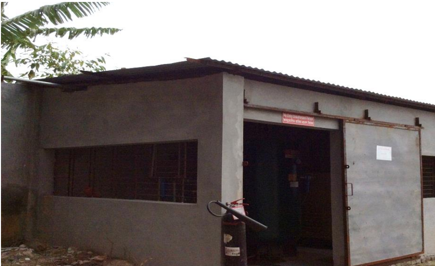
Compressor Room – Corrugated roof on steel angles
