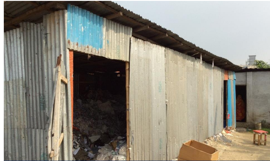
Shed 6 – Corrugated roof on timber purlins on bamboo posts
