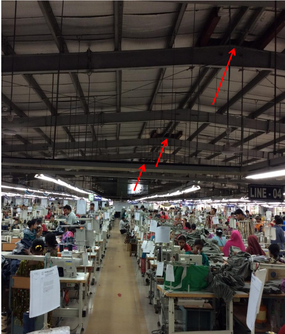
Air vents viewed from Shed 1 floor
