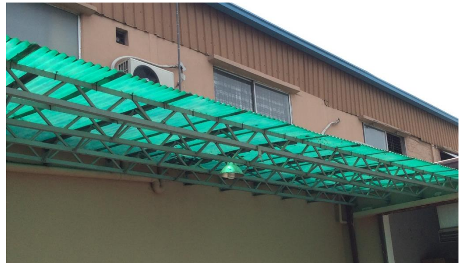
Main Entrance Canopy to Shed 2 – Corrugated plastic roof on steel angle truss
