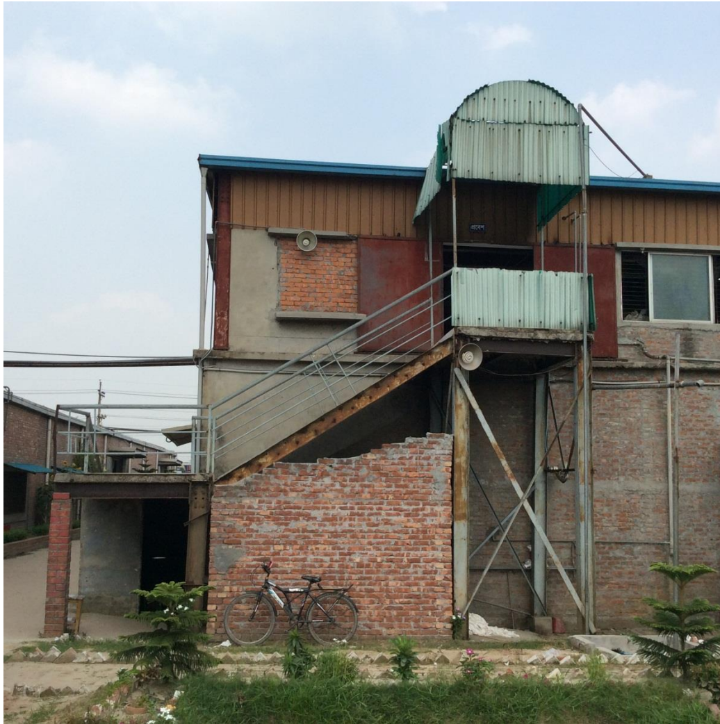
External steel stair to NW corner of Shed 2
