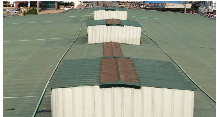
Air vents viewed from Roof
