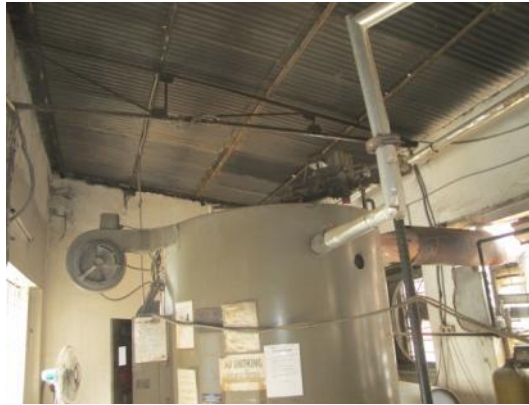
Boiler room roof structure
