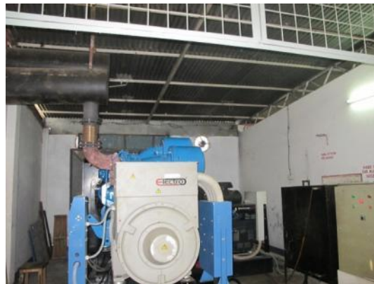
Generator room roof structure
