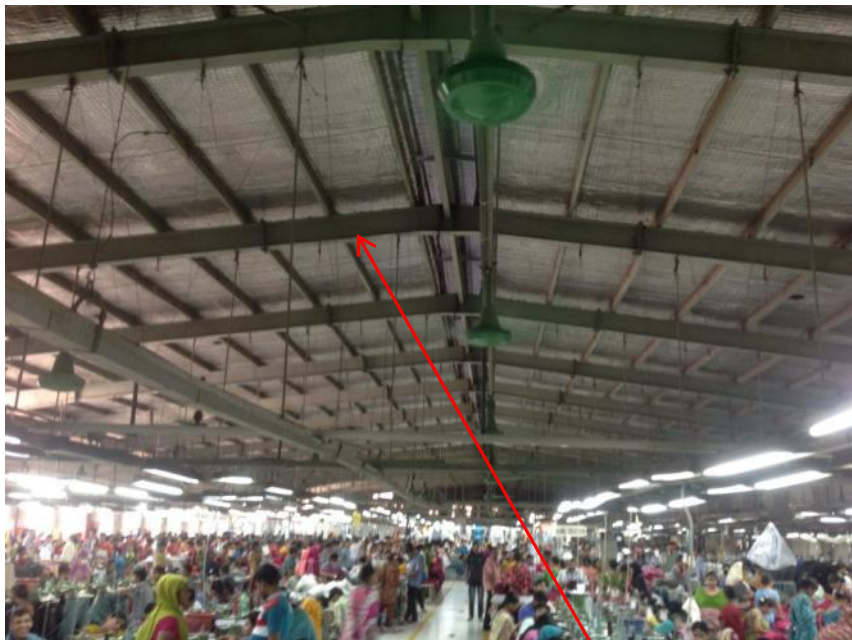
Straight rafter structure as built
