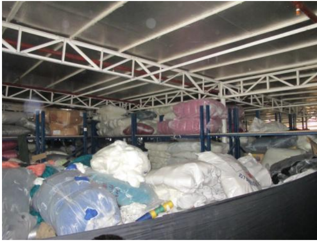
Yarn storage roof structure, some trusses supported off racking system
