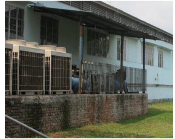
Building 2 - adjacent steel structure
