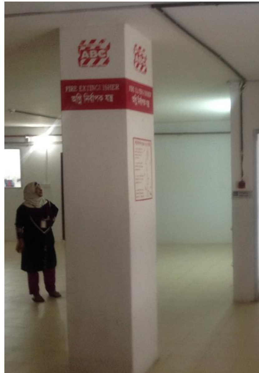
Column supporting flat slab
