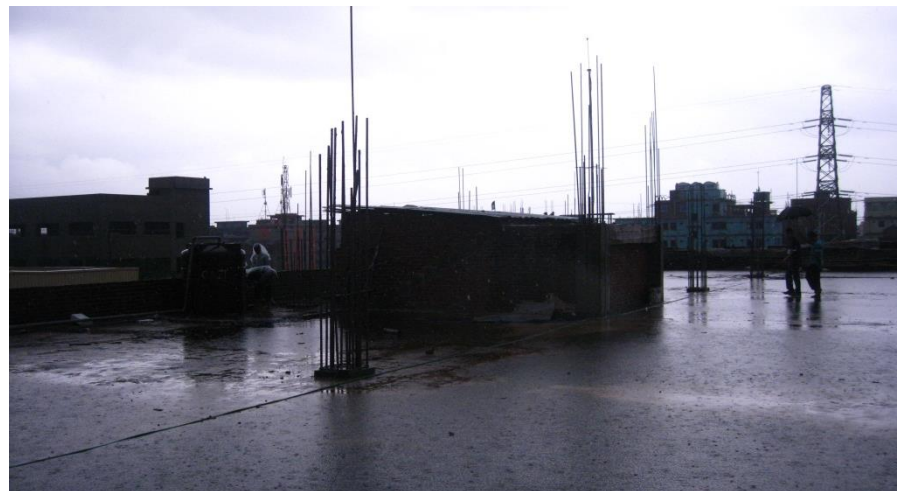
Roof to Northwest stair core
