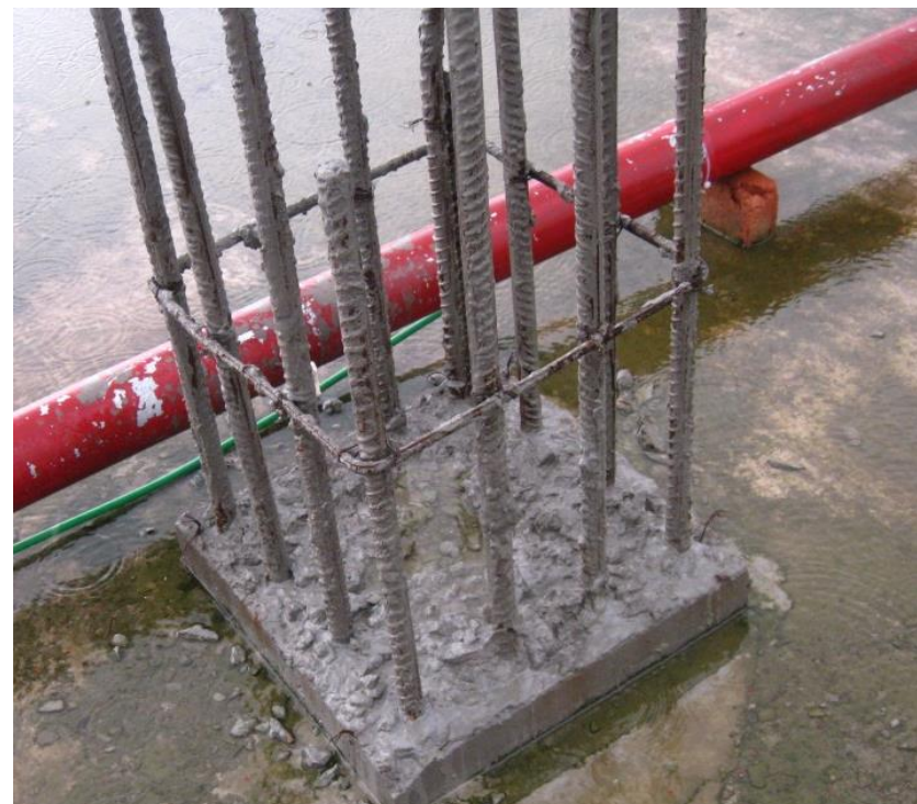
12 no. bars observed in internal column C4 at Roof level and confirmed at Ground Floor level using the Ferro-scanner
