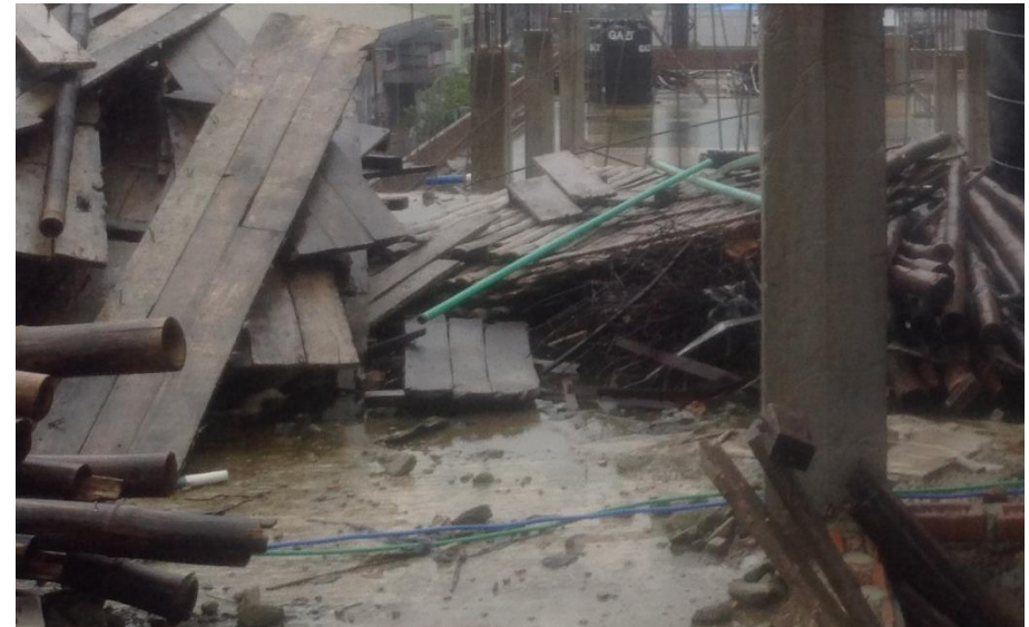
Construction materials on roof (2 nd Floor)
