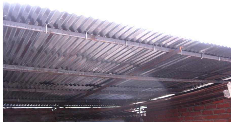
Roof to North stair core
