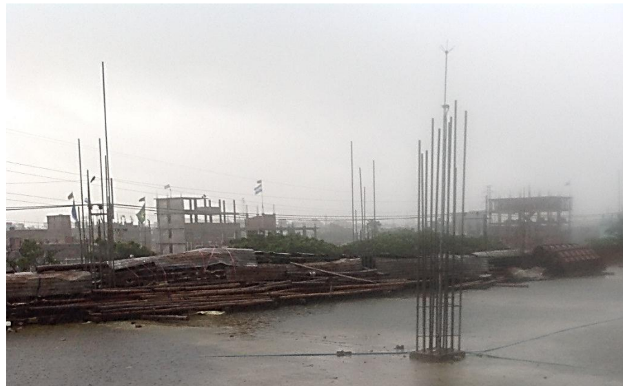
Construction materials on roof (2nd Floor)
