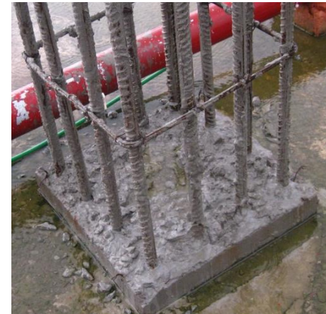
12 no. high yield rebar
