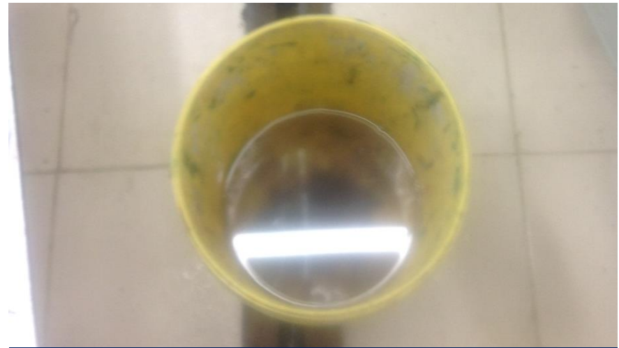
Collected water in a pail during heavy rainfall
