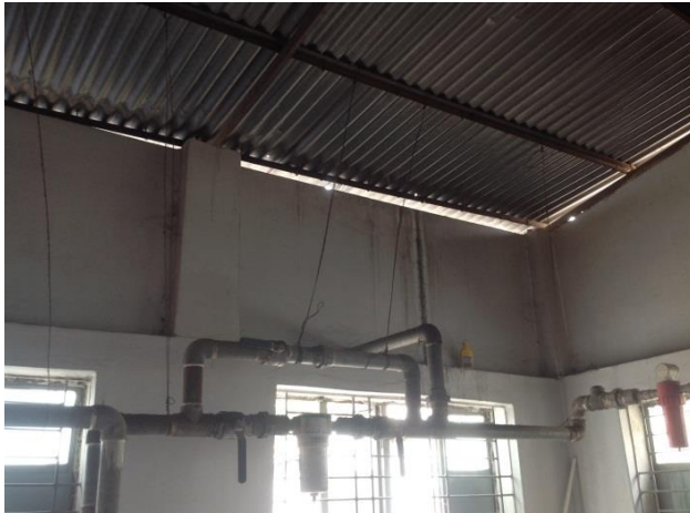
Lightweight roof to Compressor Room
