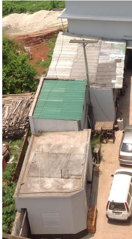
Roofs to Substation and Diesel Generator Room
