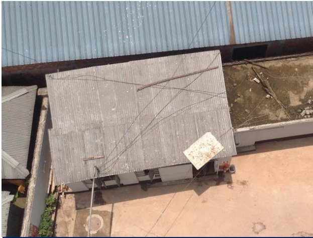
Lightweight roof to Compressor Room
