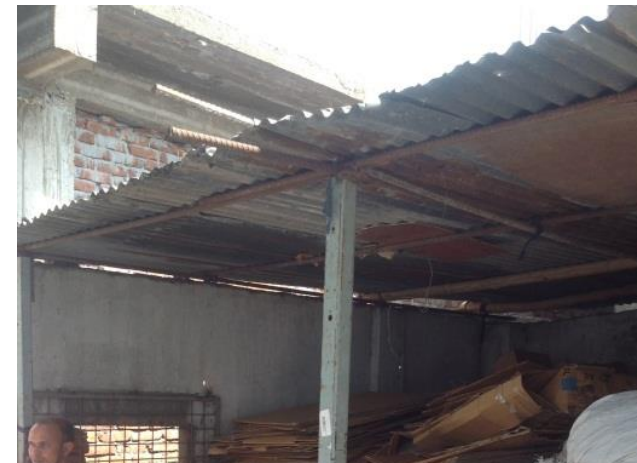
Lightweight roof to Wastage Shed
