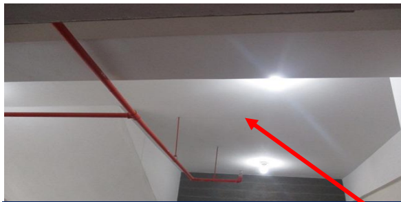
No sub beam at lift core (south)
