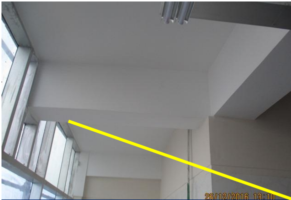
Cantilever beam at north
