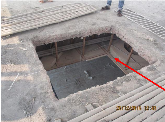
Opening in slab at 9 th floor
