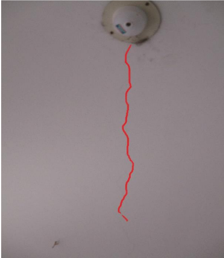
Cracking found on slabs on several panels of different floors.
