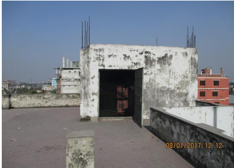
Exposed & corroded rebar found in stair case
