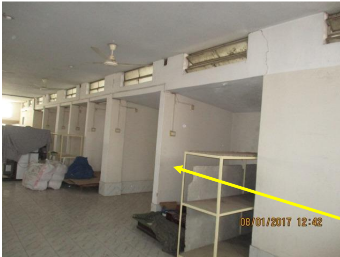
Cantilever at west with toilet area
