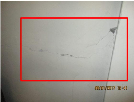
Diagonal cracks found in brick wall at 3 rd floor and below stair landing.
