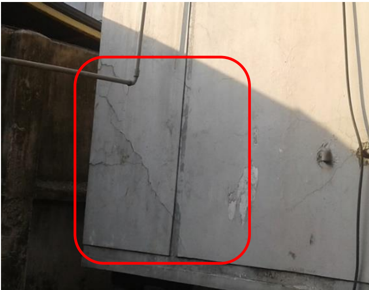
Cracks also found at south façade.
