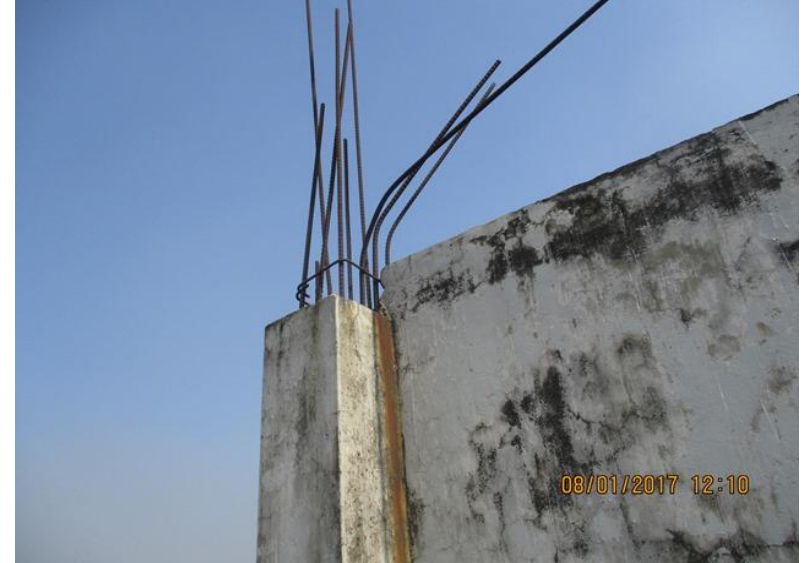
Exposed & corroded rebar found in stair case
