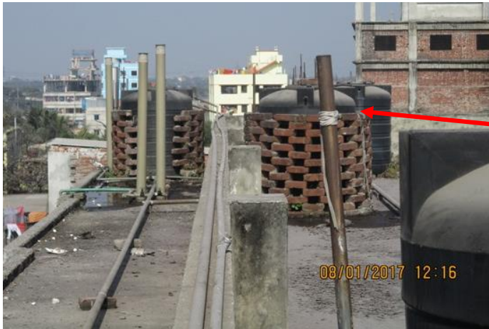
Plastic water tank on roof
