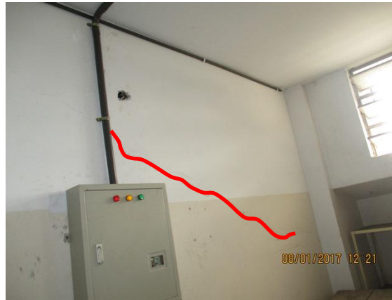
Diagonal cracks found in brick wall at 3 rd floor and below stair landing.
