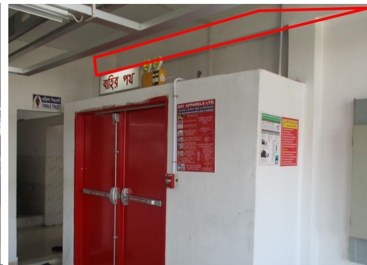
Beam was observed around stair case
