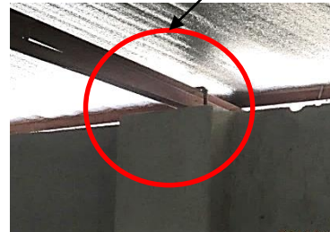
End Connection between Column and truss
