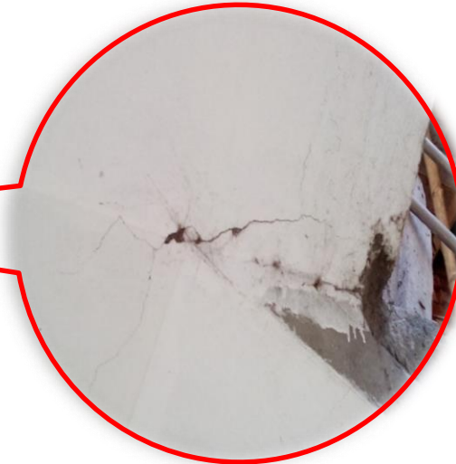
Crack observed under 3 rd floor roof slab
