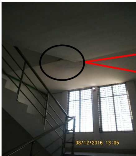
Water Dampness found on 3 rd floor roof slab on several places
