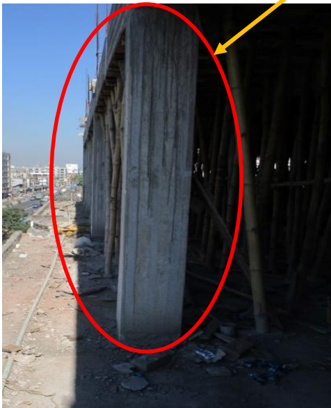
Square column 3 rd to roof top
