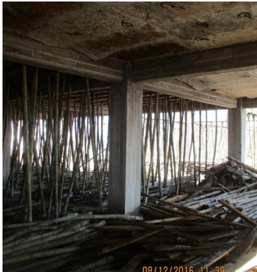
Beam under the 4 th floor top slab
