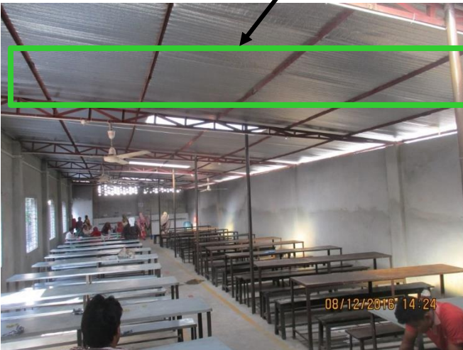
Observed seven purlin in the shed
