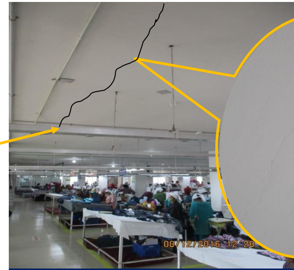
Crack observed under 3 rd floor roof slab
