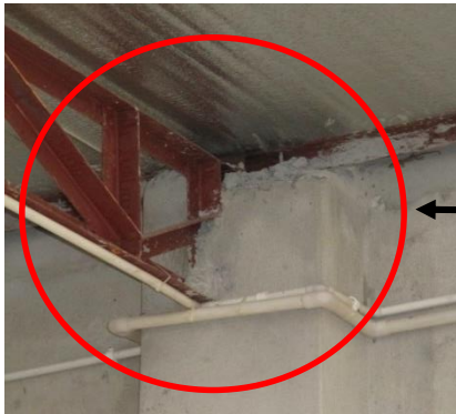
Truss connection with RC column
