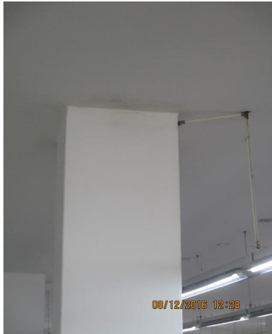
Water Dampness found on 3 rd floor roof slab on several places
