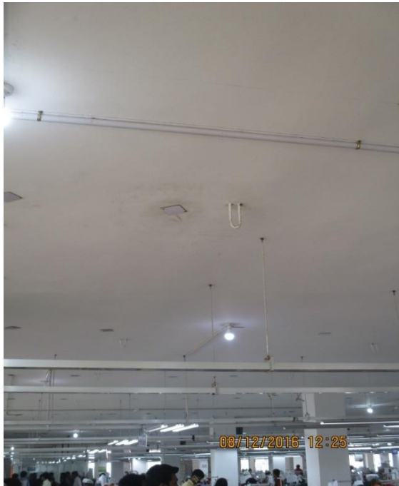
Water Dampness found on 3 rd floor roof slab on several places
