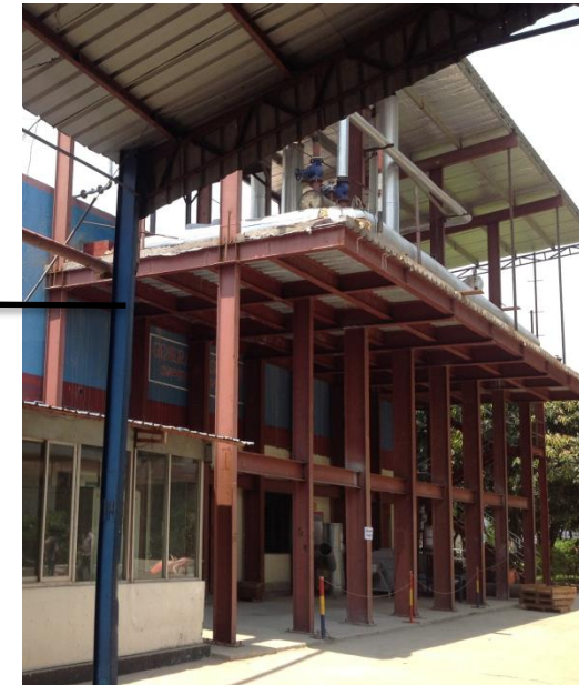
Generator & Power house extension
