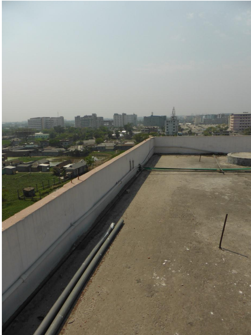
Unrestrained roof parapets
