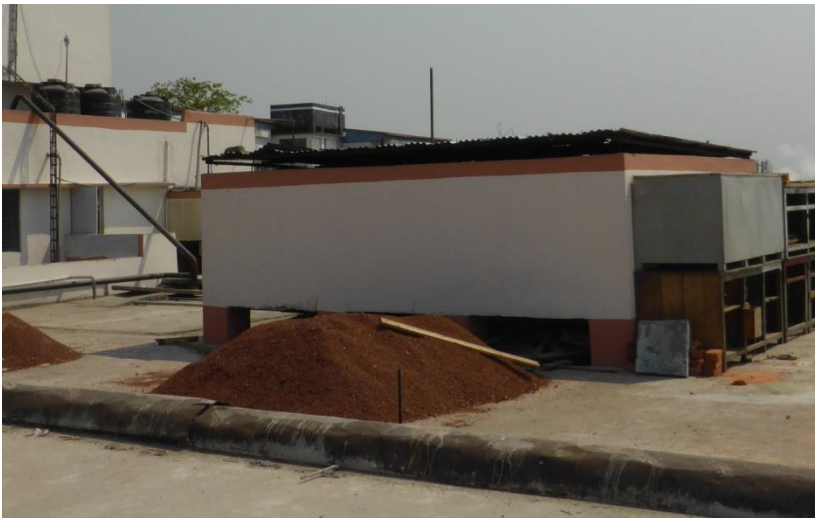
Water Tank locations at roof level and storage of aggregate.
