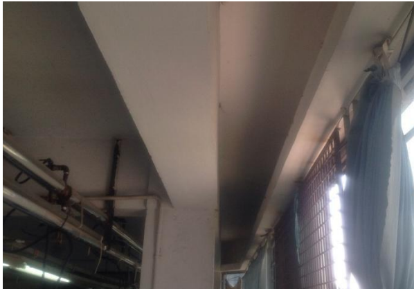
Cantilevering slab to East elevation
