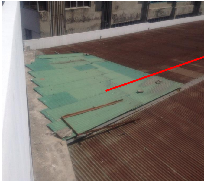
Remedial Works to Steel Roof
