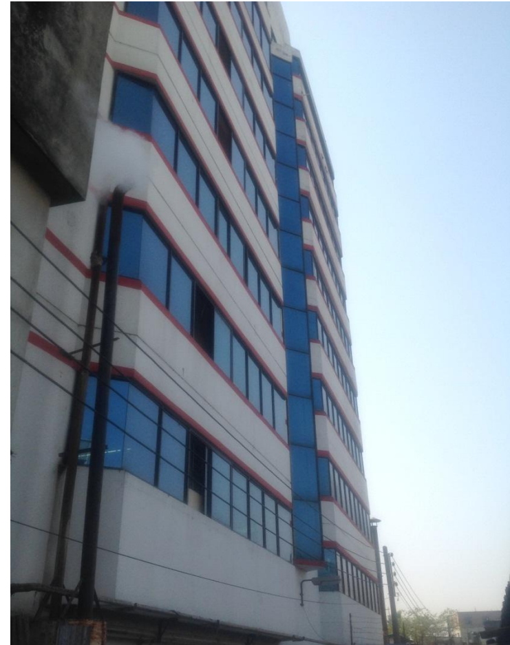
View of Façade to East Elevation
