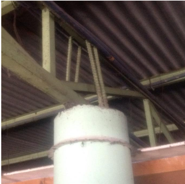
Steel Roof Column Connection
