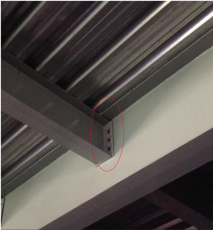
Slotted bolt holes
