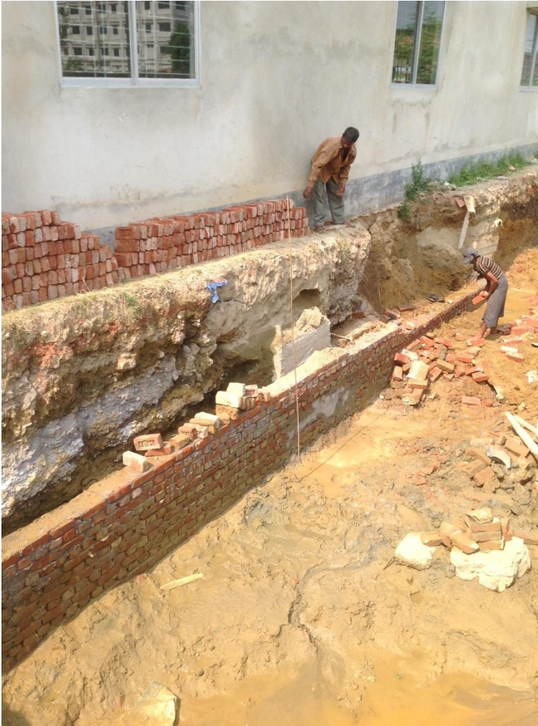
Exposed pad footing under edge column
