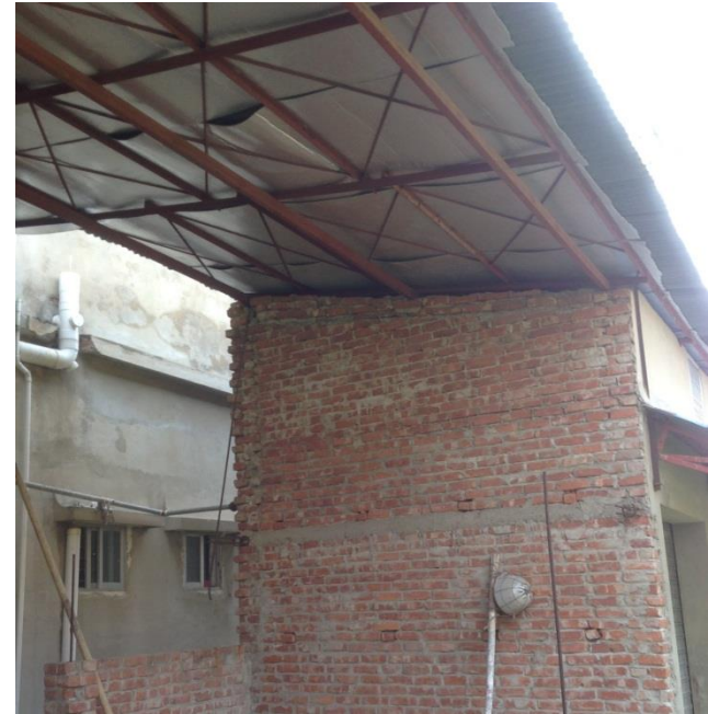
Ancillary plant building roof
