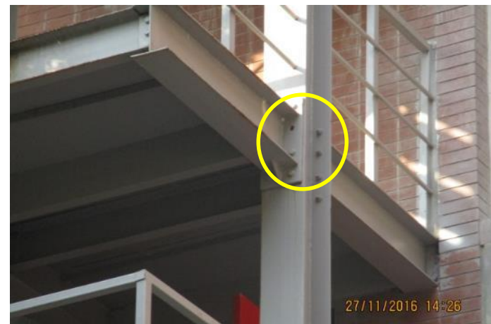
Stair at utility building
