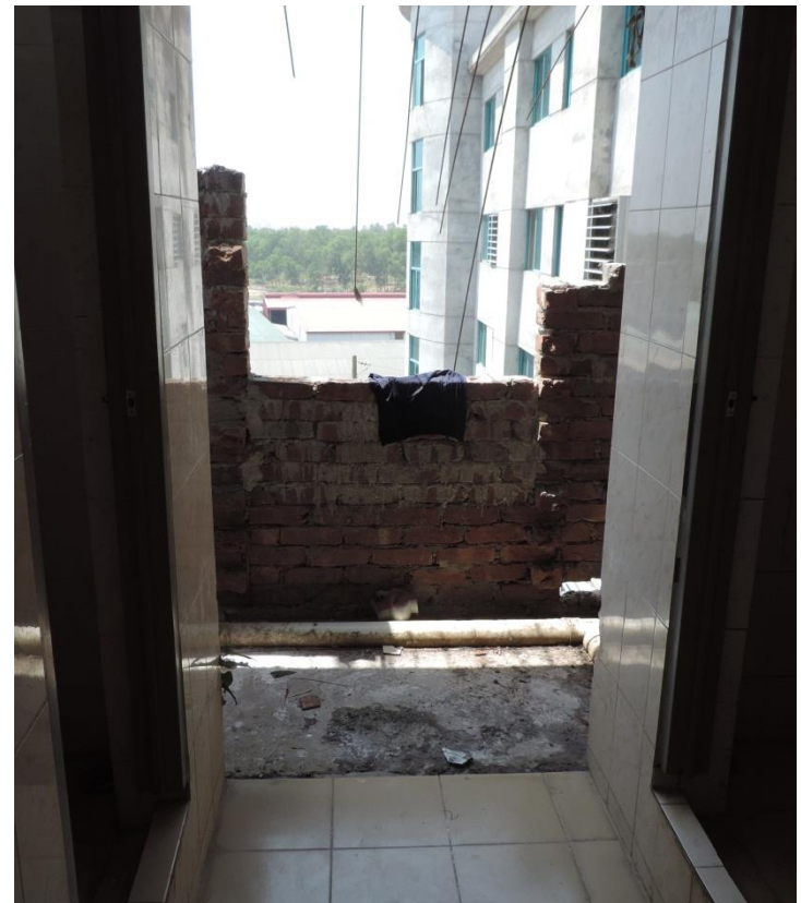
View from inside male toilets
