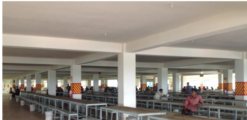
Typical beam and slab structural system
