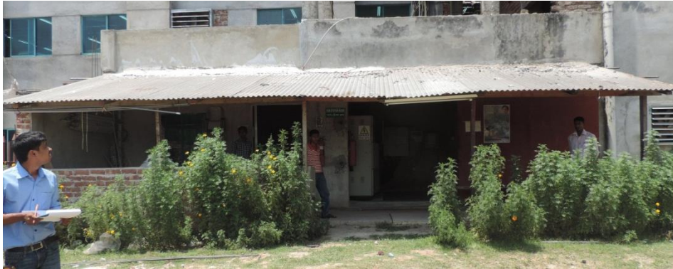
Single-storey generator room
