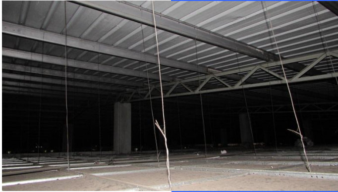
New steel roof
