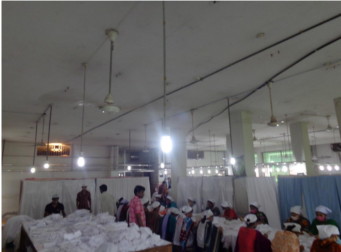
No beams between the columns (flat slab construction)
