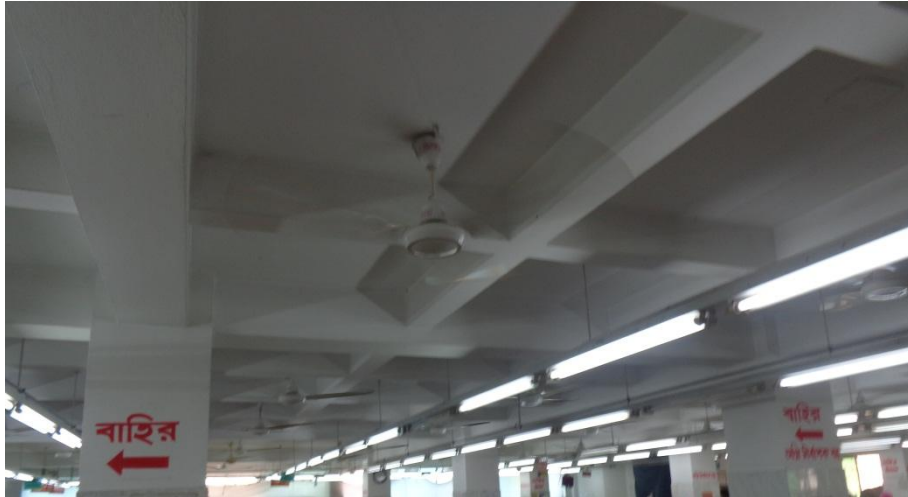
Underside of 3 rd Floor Slab
