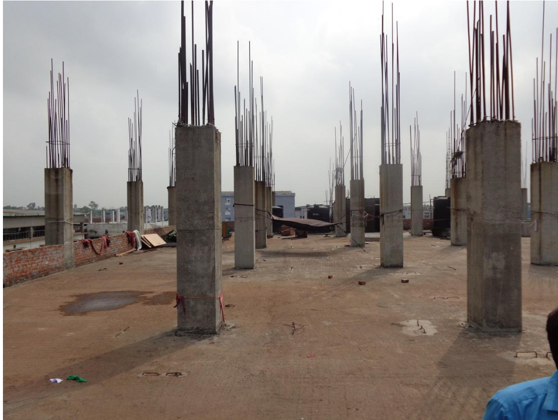
5 th Floor/Current Roof Level
