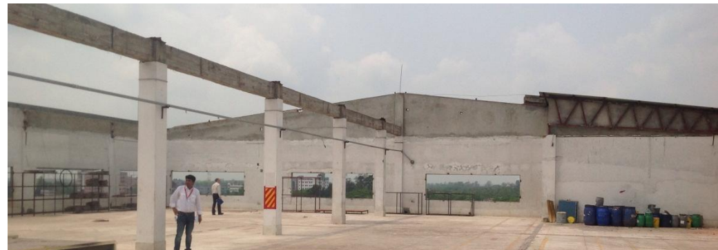
5m high wall to perimeter of Roof level
