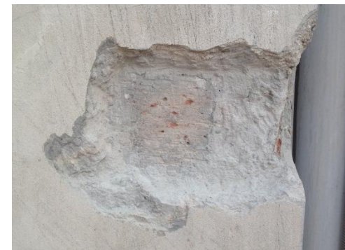
Tested Column E/1 (Brick)
