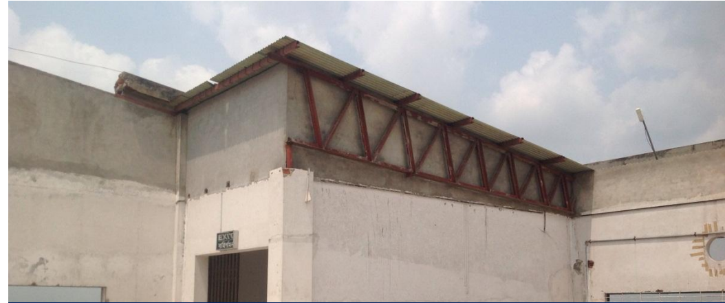
Lightweight Roof to Staircore
