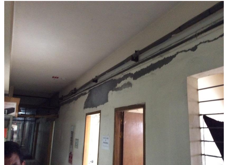
Numerous examples of cracking and evidence of repair to cracking
