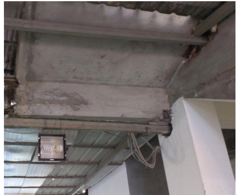
Photo taken of stairwell column as built
