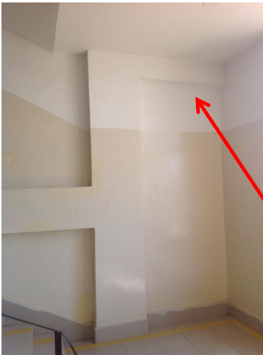
Stairwell cantilever beam
