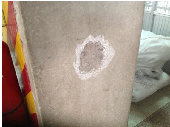
Tested Basement Column 8 Storey Building – Stone Chips
