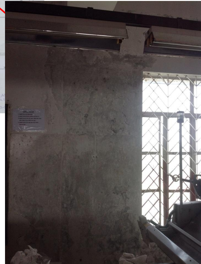
Water ingress on 4 th floor of 6 storey building
