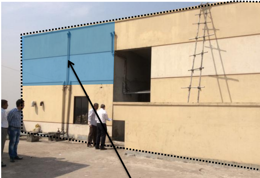
Water tank height 2.3m over bay of stair core = 23kN/m 2
